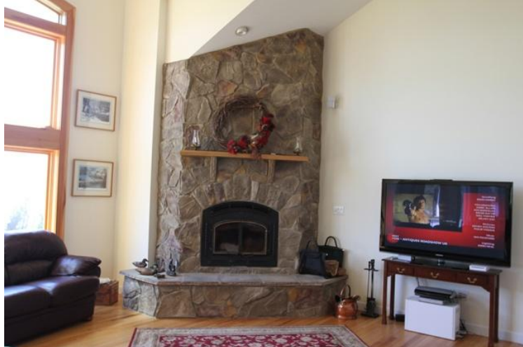
Figure 16. First floor fireplace in great room. Note continuation of void space to left of fireplace. Also note angled void space above fireplace.
