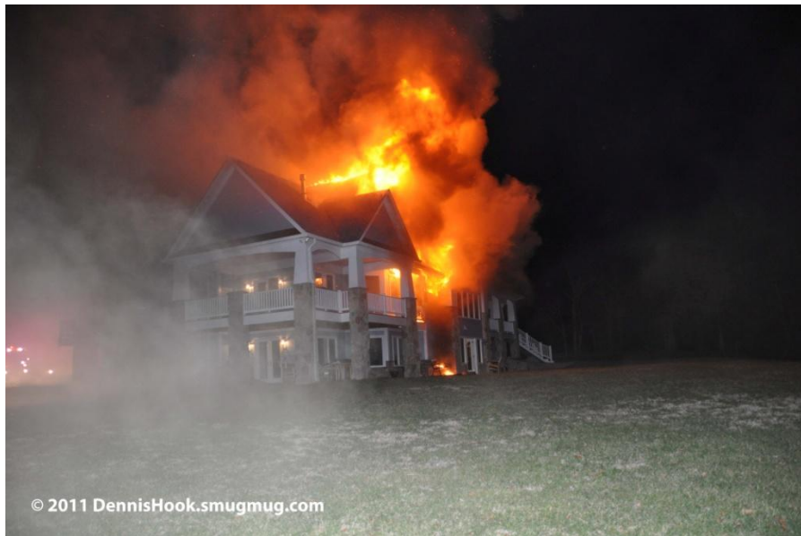
Figure 25. Photo of Side Charlie prior to the event on the second floor. Note that the main body of fire appears to be coming from the attic, gabled void space above the great room.
