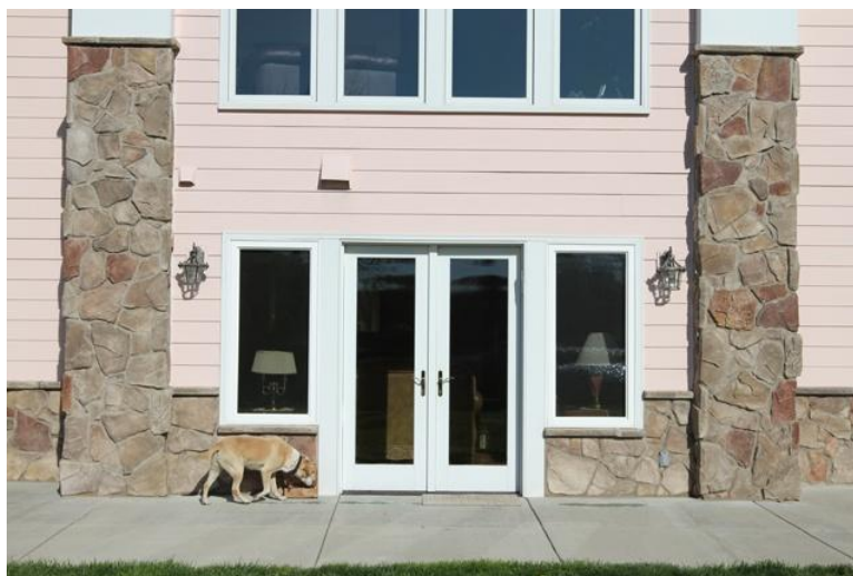
Figure 15. Close-up of basement living area door. Note stone veneer columns.
