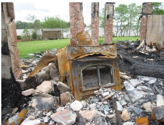
Figure 19. Basement living area fireplace. Note hole on left side of fireplace and outer edge of stone veneer of void space.
