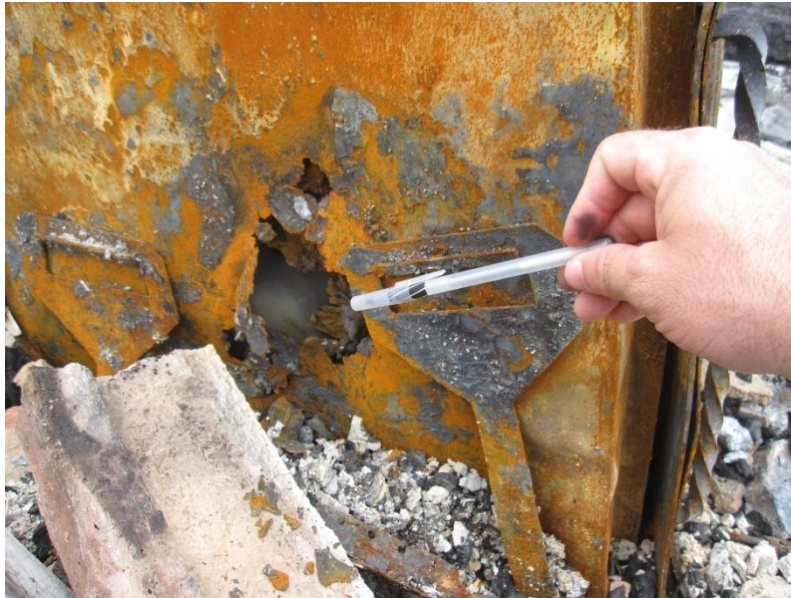
Figure 21. Corrosion hole in fireplace.
