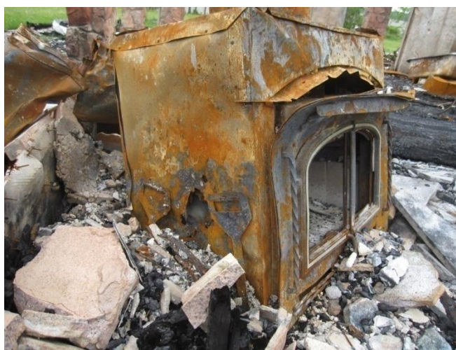
Figure 20. Close up of fireplace. Note corrosion hole in left side of fireplace.
